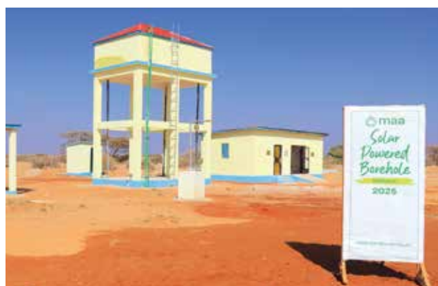
Muslim Aid Australia funded a new borehole in Banadir in 2025, providing clean water to 18,000 people
