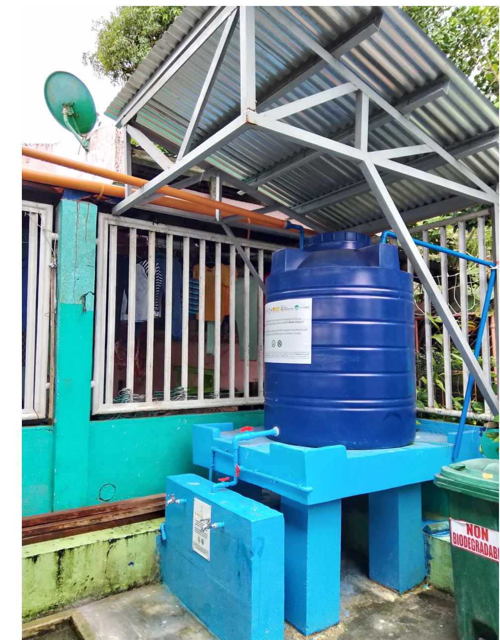
Rainwater harvesting installed in a barangay (village) in The Philippines based on NEAT+ recommendations
