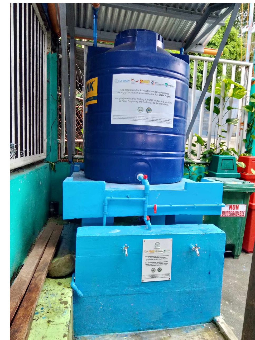
Rainwater harvesting installed in a barangay (village) in The Philippines based on NEAT+ recommendations
