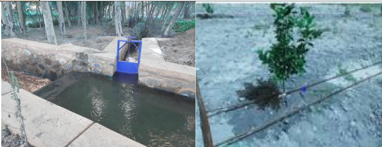
Figure 2: Effective irrigation systems promoted by DACAAR
